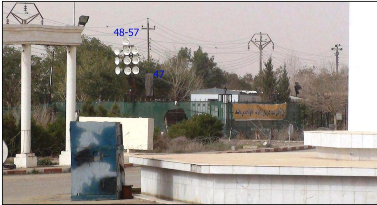
Eleven loudspeakers, installed right on top of the hospital entrance gate (Main entrance at Ashraf's western flank)
